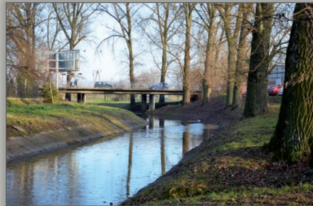
Most na rzece Plonce Bridge over the river Plonka
